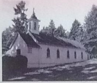
St. Peter (1863) 910 South Street, Suquamish
