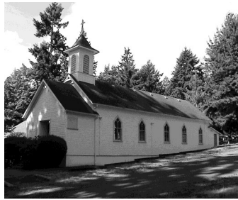
St. Peter (1863) 910 South Street, Suquamish
