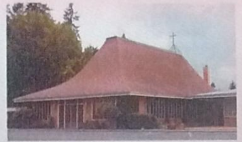
St. Olaf (1968) 18943 Caldart Ave. NE, Poulsbo, 98370
