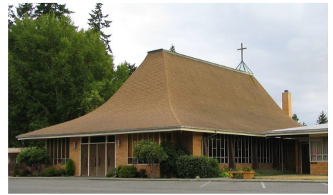
St. Olaf (1968) 18943 Caldart Ave. NE, Poulsbo, 98370
