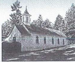
St. Peter (1863) 910 South Street, Suquamish
