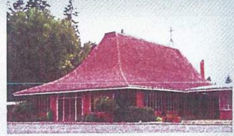
St. Olaf (1968) 18943 Caldart Ave. NE, Poulsbo, 98370
